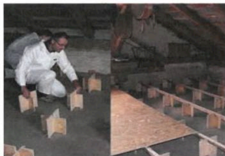
pose double plancher
